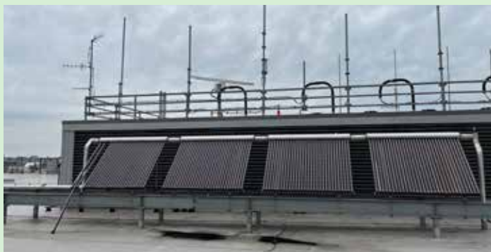
Evacuated tube solar collectors on the roof of Terminal B's Arrivals and Departures Hall help reduce natural gas consumption.
